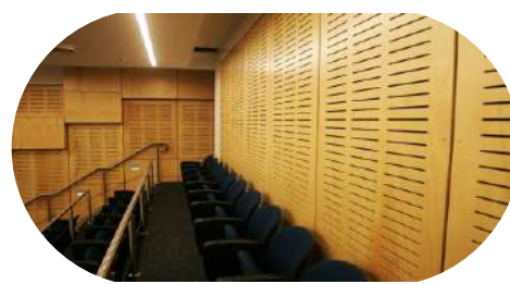
MODEL : SLT-P SIZE : 600X600/1200X16/17 MM SLIT PERF.: 10X75 MM
